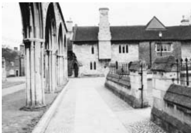
Positive features of the conservation area: the Infirmary Arches.
