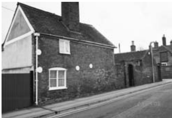
No. 14 Pitt Street is a modest unlisted building that is important in establishing the building line and the key architectural themes for the eastern stretch of Pitt Street.
