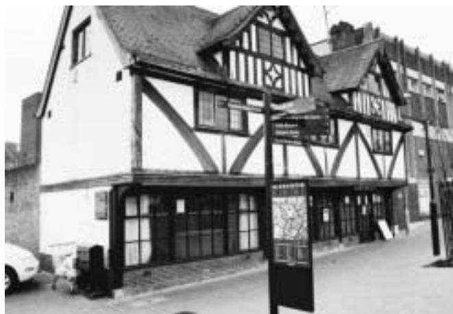
Built as an inn in the sixteenth-century, the Raven Centre lies along the line of a major historic route into and out of Gloucester.
