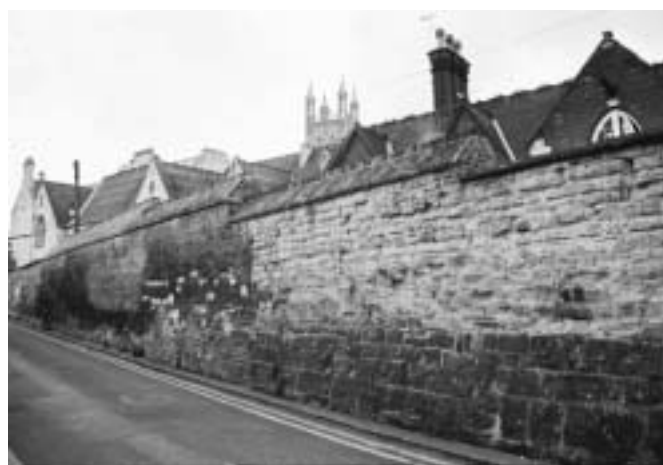
To a large extent, the boundaries of the conservation area are defined by the walls of the medieval abbey.
