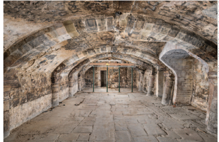
The 12th Century undercroft in the Grade I listed Fleece Hotel
