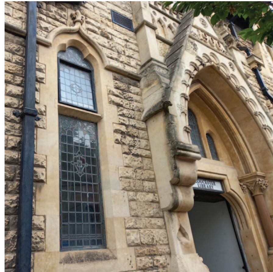
Victorian gothic details on the Public Library, Brunswick Road
