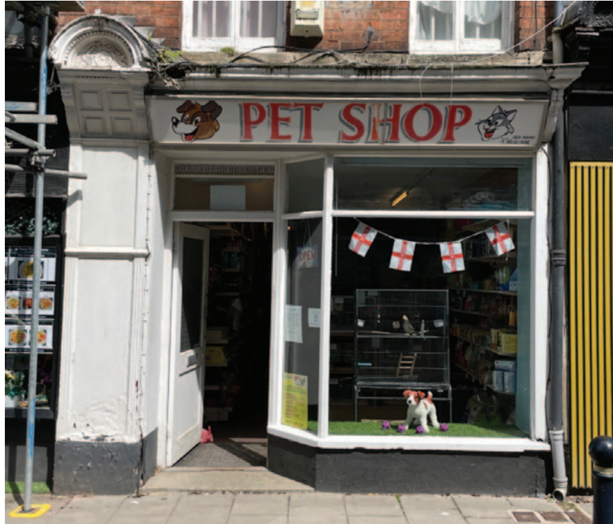
Historic shopfront on St.Aldate
