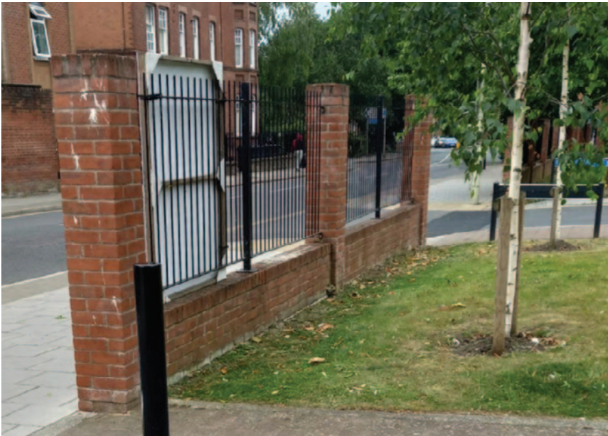
Boundary treatments in the Brunswick Road, Greyfriars and Eastgate Character Area
