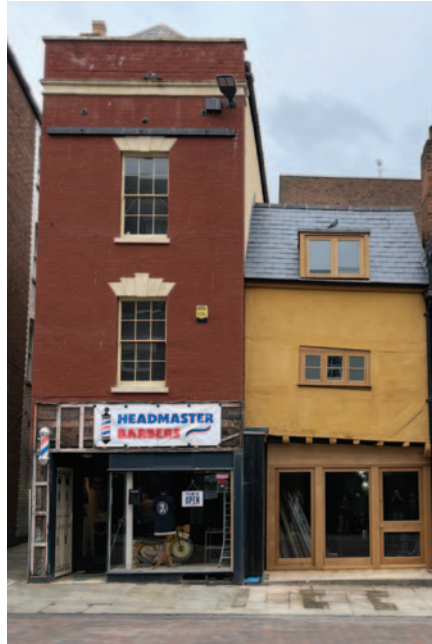
16th century timber framing (right) and 19th century brick façade (left) at 39-41 Westgate Street – both Grade II listed buildings
