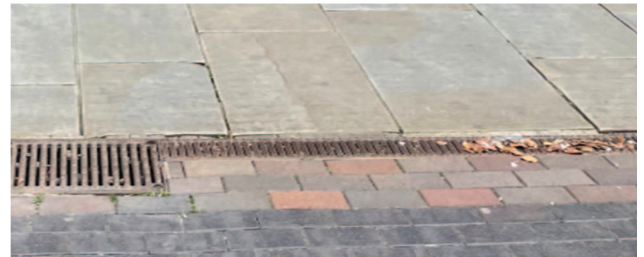
Street surfaces in the Gate Streets Character Area
