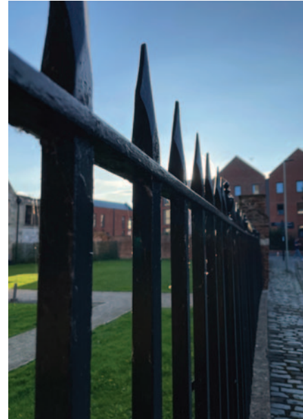
Boundary railings at Blackfriars
