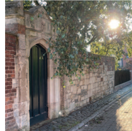
Historic boundary wall at Blackfriars
