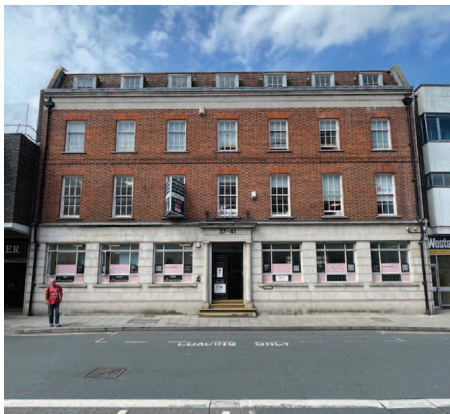
Nem House, Clarence Street
