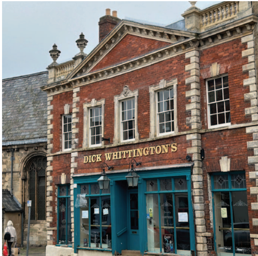
Grade I listed Dick Whittington's (100 Westgate Street)
