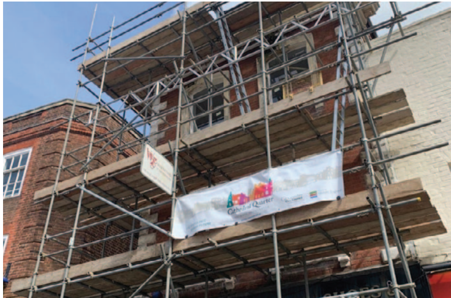
Works at 14 Westgate Street as part of Gloucester HSHAZ
