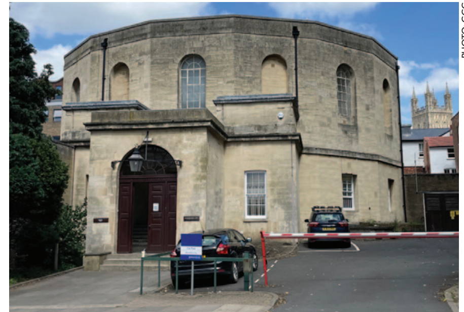
Gloucester Crown Court
