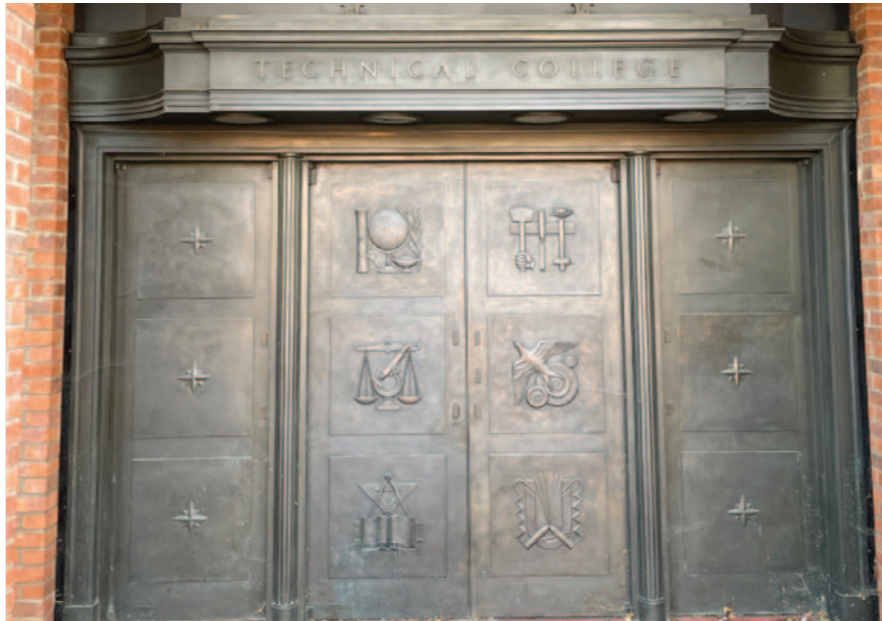
The cast bronze doors of the now demolished Technical College, preserved as part of the Friars Orchard development.
