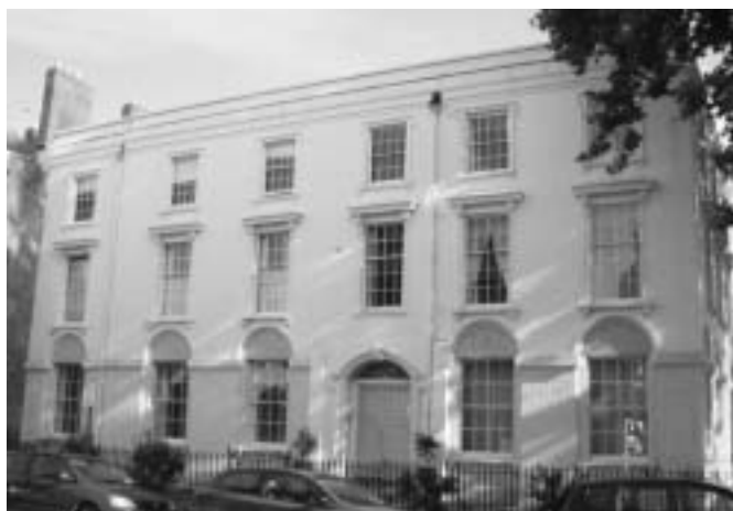
The former Spa Hotel, Spa Road.
