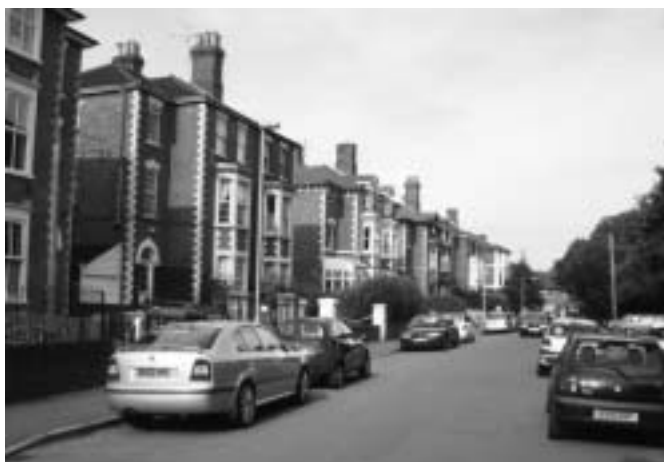
Weston Road (south side).
